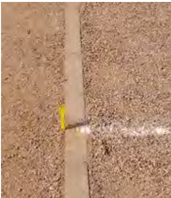
↑ Use of landscape blocks for shooting lines. PASEO VISTA RECREATION AREA , Chandler, Ariz.
